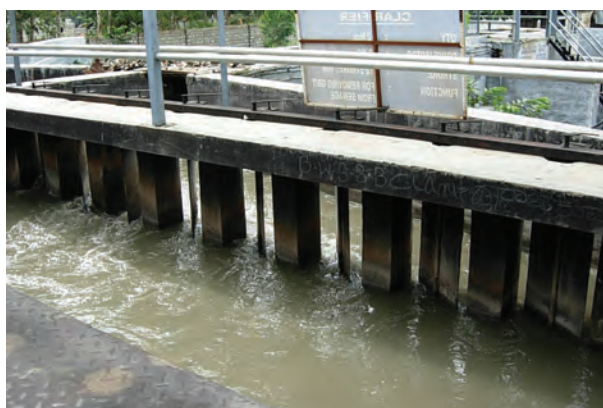
Fig. 13.4 Grit and sand removal tank
